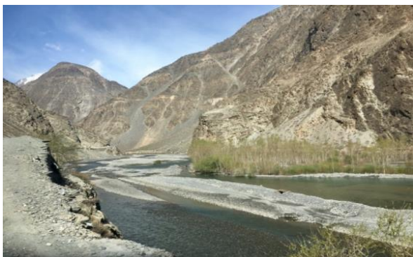
Fig. (3). Unstable roads in the mountainous region of Chitral.
